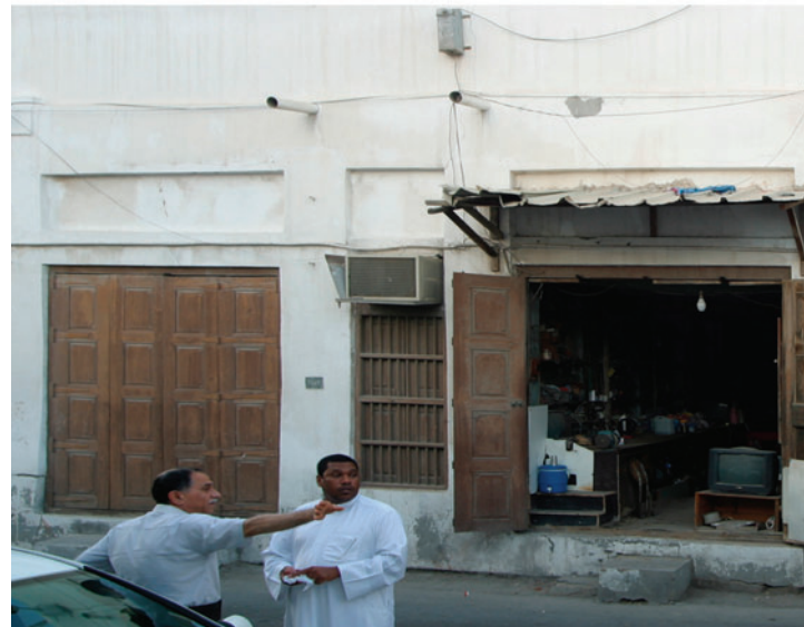
Rectified photograph of the same storefront. Rectification removes perspective, angle, and camera lens distortion to create an image that is on one plane and measurable. Photo: © Salim Elwazani and José Luis Lerma.
