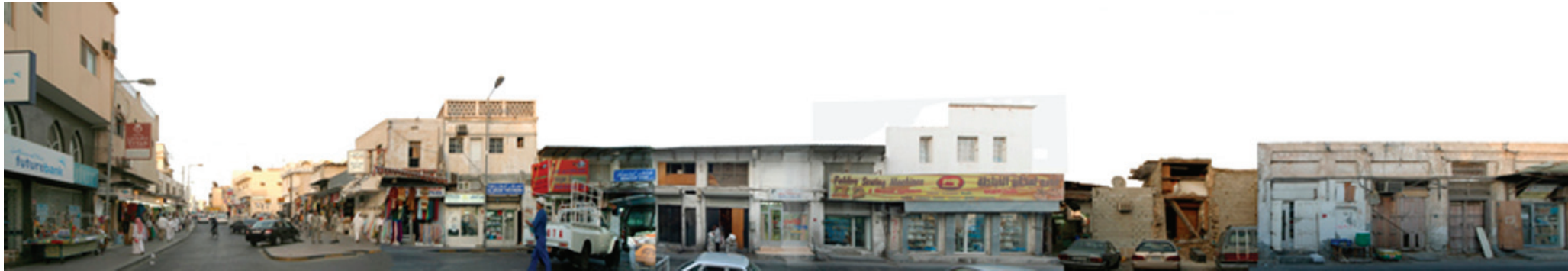
Mosaic of Souq West elevation on Tujjar Street. Photos: © Salim Elwazani and José Luis Lerma.
